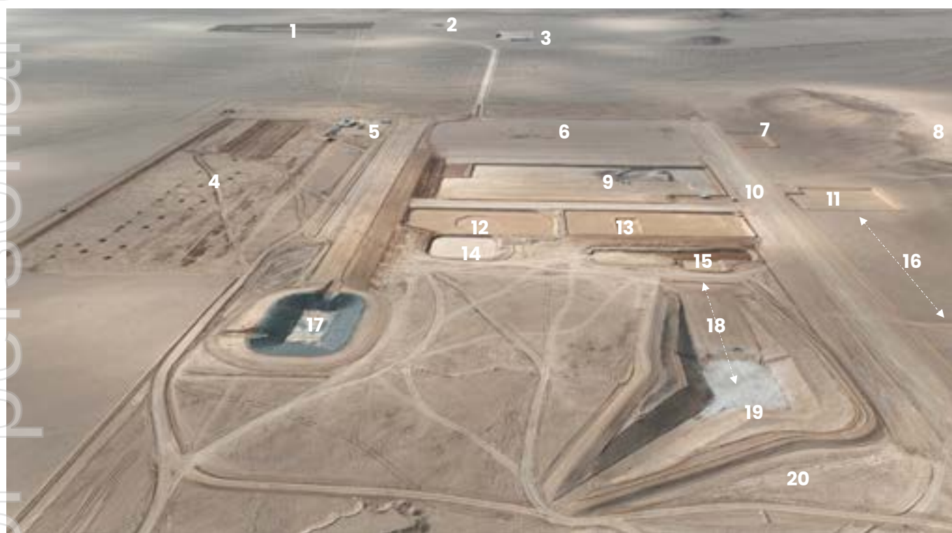
Figure 2: Aerial view of the Tumas Project bulk earthworks May 2026
