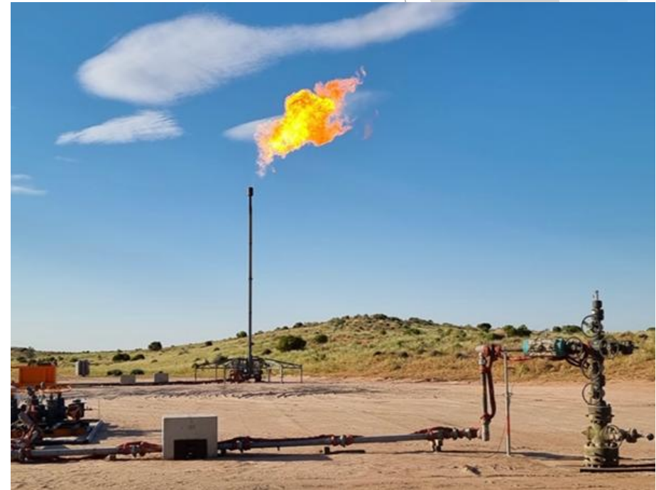
Gas flare at Kiwi-1 wellsite
