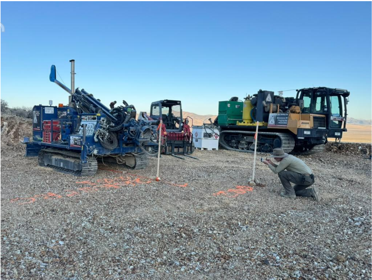
Figure 1: RC Drill rig successfully mobile to the Keystone Project, Nevada
