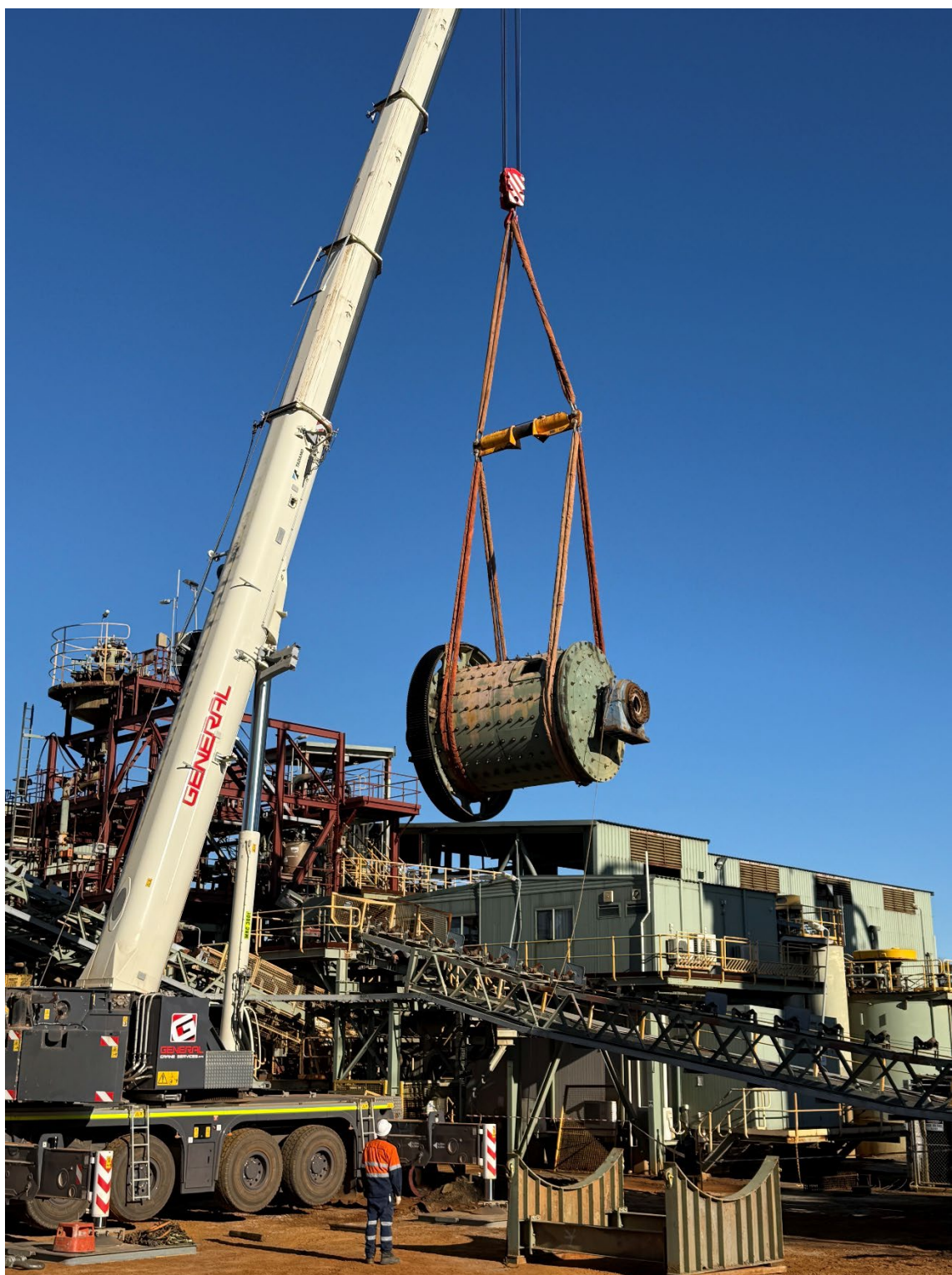
Image 1: Mill Refurbishment significantly advanced
