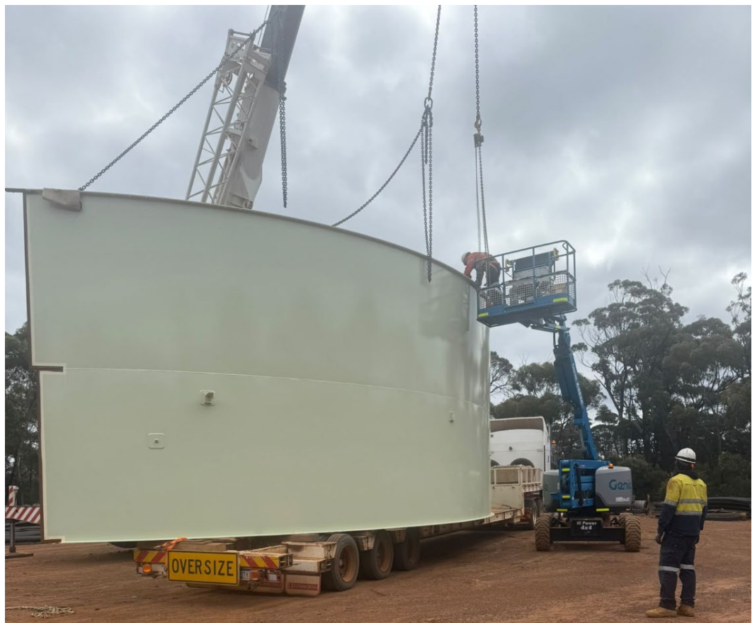
Image 4 & 5: Lake Johnston Processing Facility – CIL tank sections
