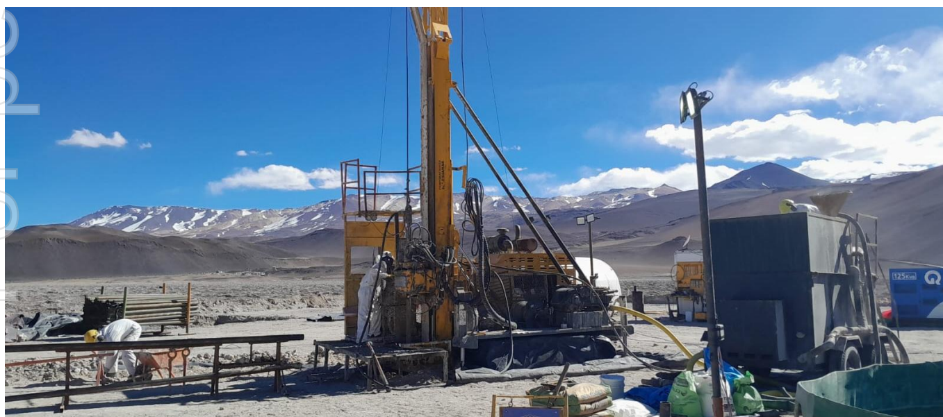
Figure 1 – DDH-4 underway at the Demasia tenement
