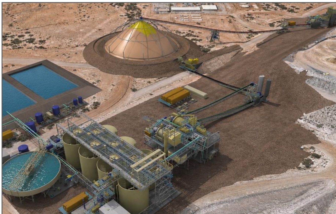
Figure 3: Mt Magnet Circuit 2 plant layout
