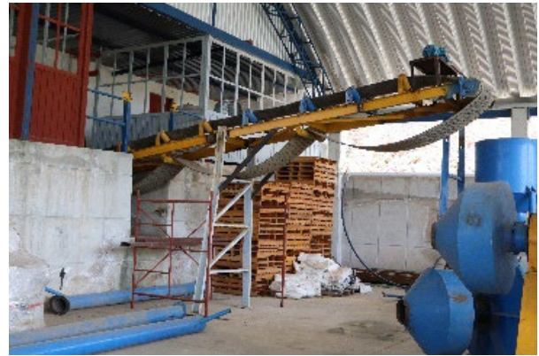
Figure 3: Mill feed conveyor installation
