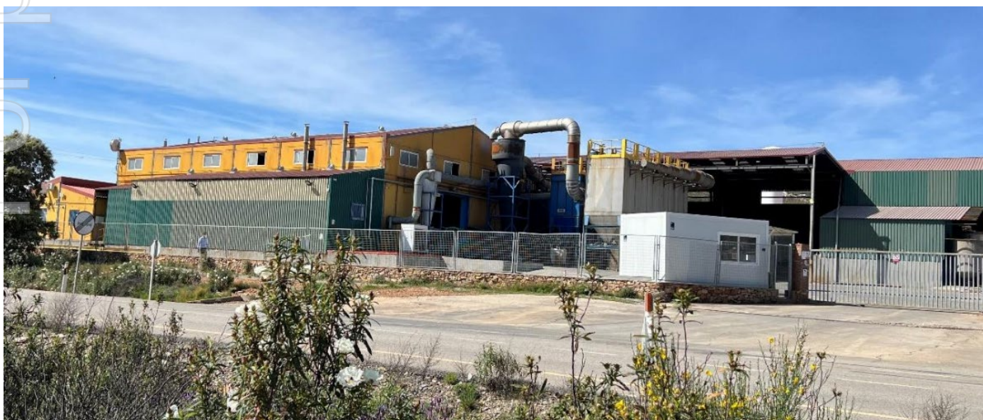
Figure 1. Partial external view of the Robledollano tin smelting and refining facility.
