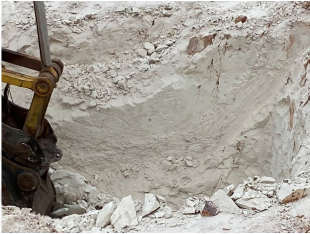
Figure 3: White Kaolin being excavated from the test pit
