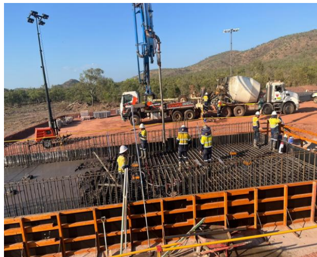
Figure 3: Process Plant Civil Works at Sorby Hills
