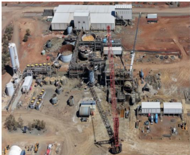
Figure 2: DeGrussa Process Plant Disassembly.
