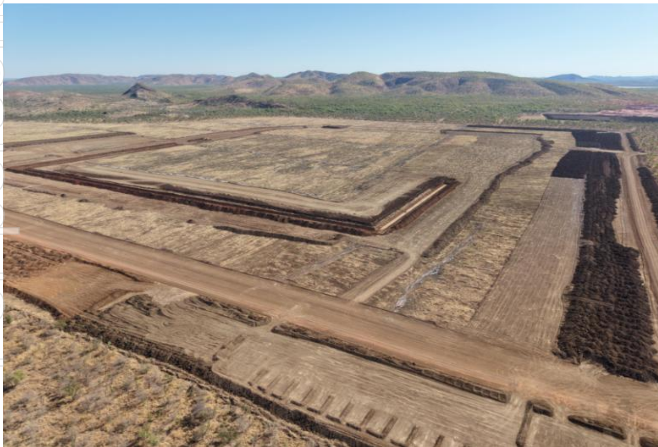
Figure 1: Tailings Storage Facility (TSF) construction at Sorby Hills
