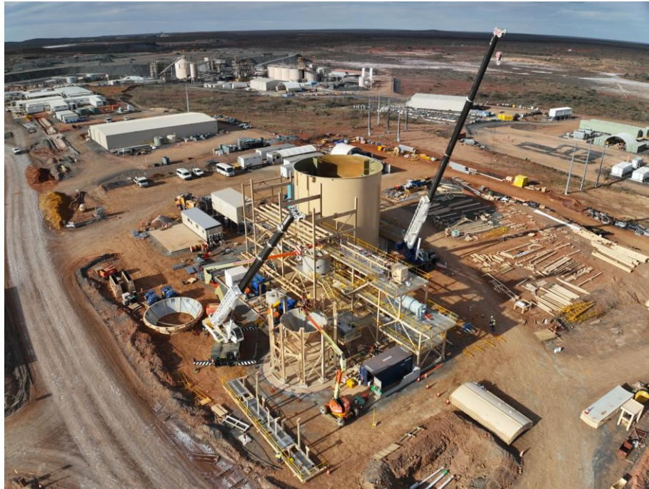
Figure 2: Paste Plant construction – October 2026.
